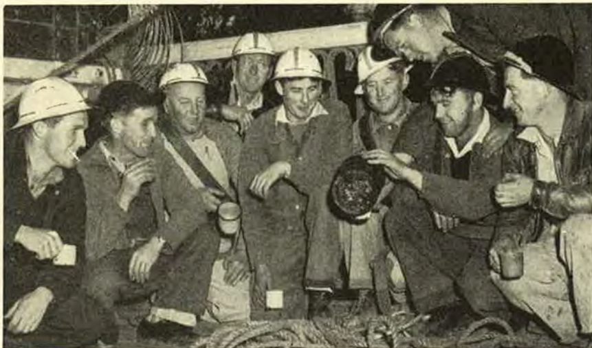
No. 1 Construction gang has a break from running a new low-tension line on the outskirts of Castlemaine. Enjoying a well-earned cup of tea despite the rain
