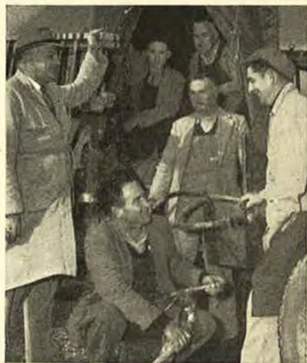
Foreman Les Atkins with construction workers J. Kennedy, R. Harrison, A. Hunter and, in truck, G. Wardley and W. McConnell, who started with the old Castlemaine electricity Supply Company.
